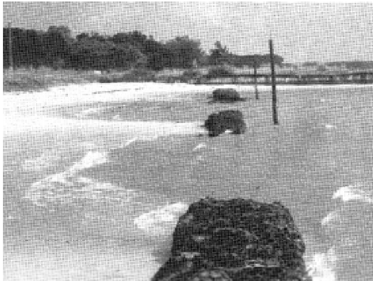
Gabions used to construct a gapped breakwater system.
