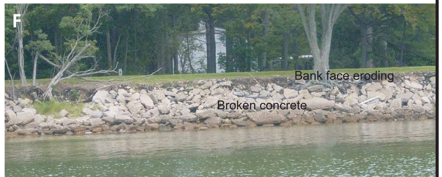
Figure 6-4. The northwest side of Gwynn's Island has many types of structures for shore stabilization A) bulkheads, B) groins and revetments, and C) riprap. In addition, along the main road onto Gwynn's Island broken concrete and poured concrete have been dumped along the shore in order to protect the road.
