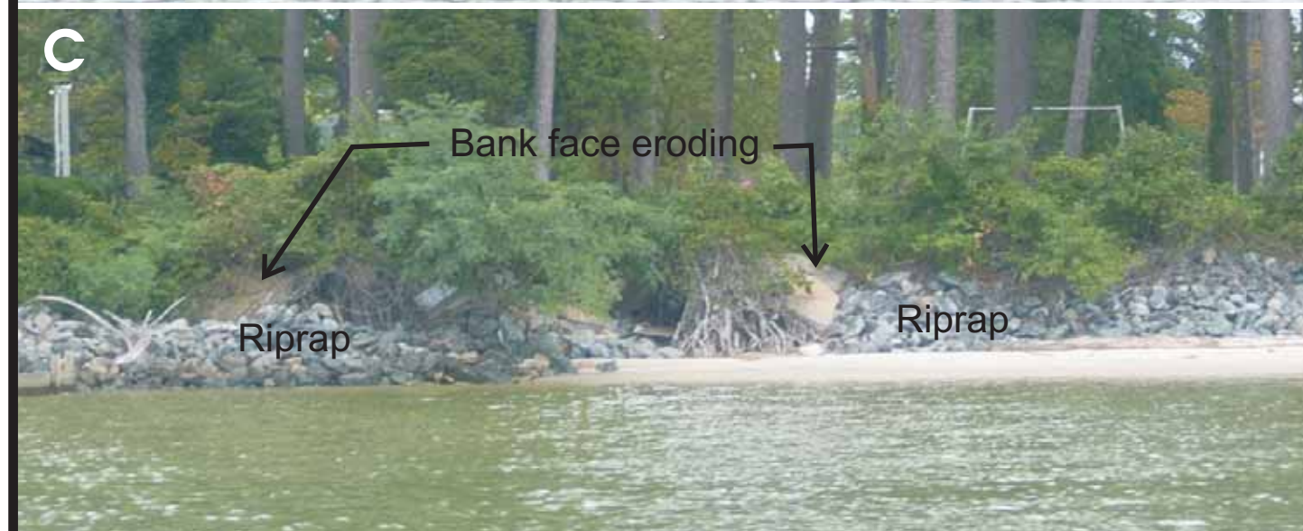
Figure 6-4. The northwest side of Gwynn's Island has many types of structures for shore stabilization A) bulkheads, B) groins and revetments, and C) riprap. In addition, along the main road onto Gwynn's Island broken concrete and poured concrete have been dumped along the shore in order to protect the road.
