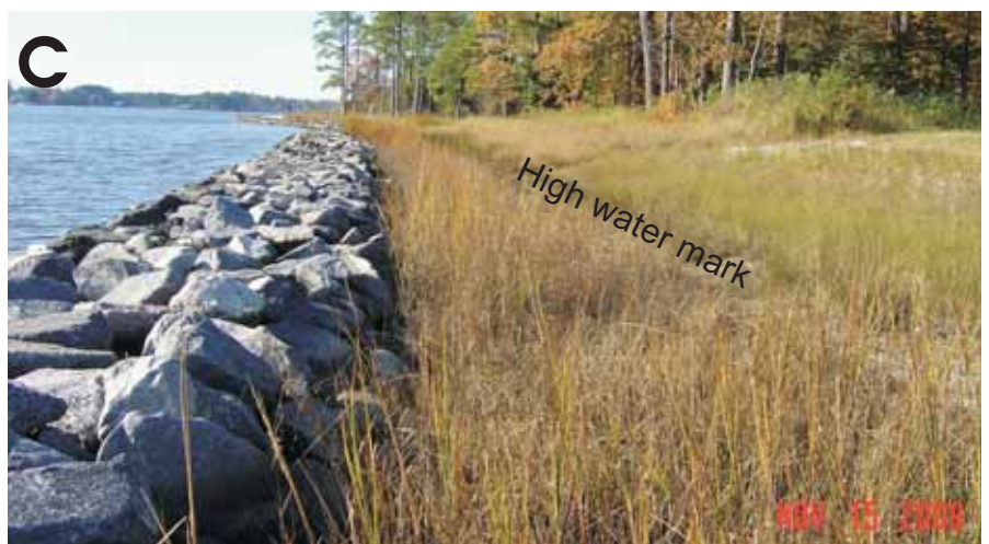
Figure 3-7. Impacts of the Veteran's Day Northeaster along select Mathews County shoreline. A) Profile data taken along the southern end of Bavon Beach showed that the beach had a large amount of erosion. B) Structures along Gwynn's Island failed and the shoreline eroded. C) A sill on the East River had no significant impact from the increased water levels and waves.
