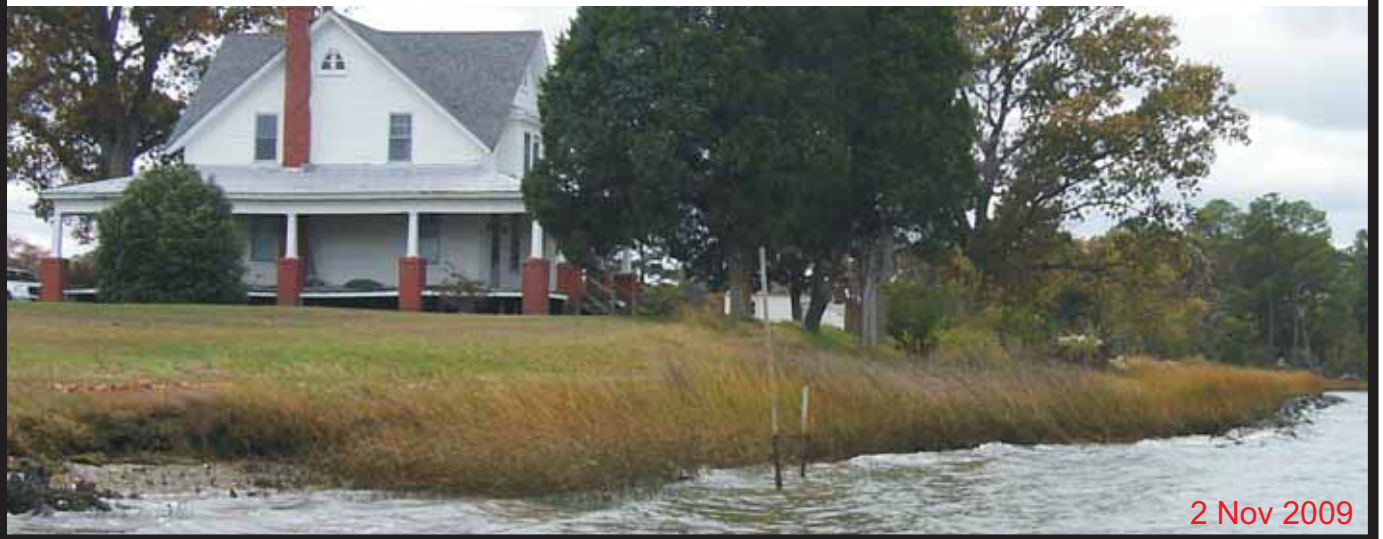
Figure 7-5. “Granddaddy sill” along the East River. Anecdotal evidence suggests this structure was placed along the shore in the late 1800s. Since that time, it has maintained the fringe marsh in front of the upland.
