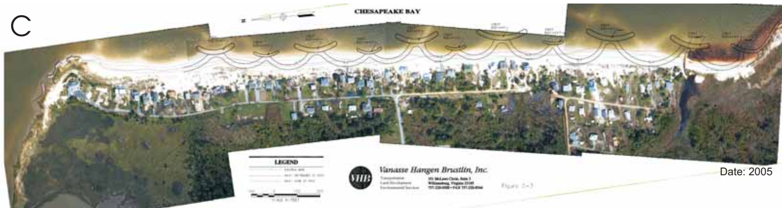
Figure 6-7. Chesapeake and Bavon Beaches showing A) extensive dune fencing, B) an alongshore view looking south toward New Point Comfort, and C) The stabilization plan developed for this shoreline reach.
