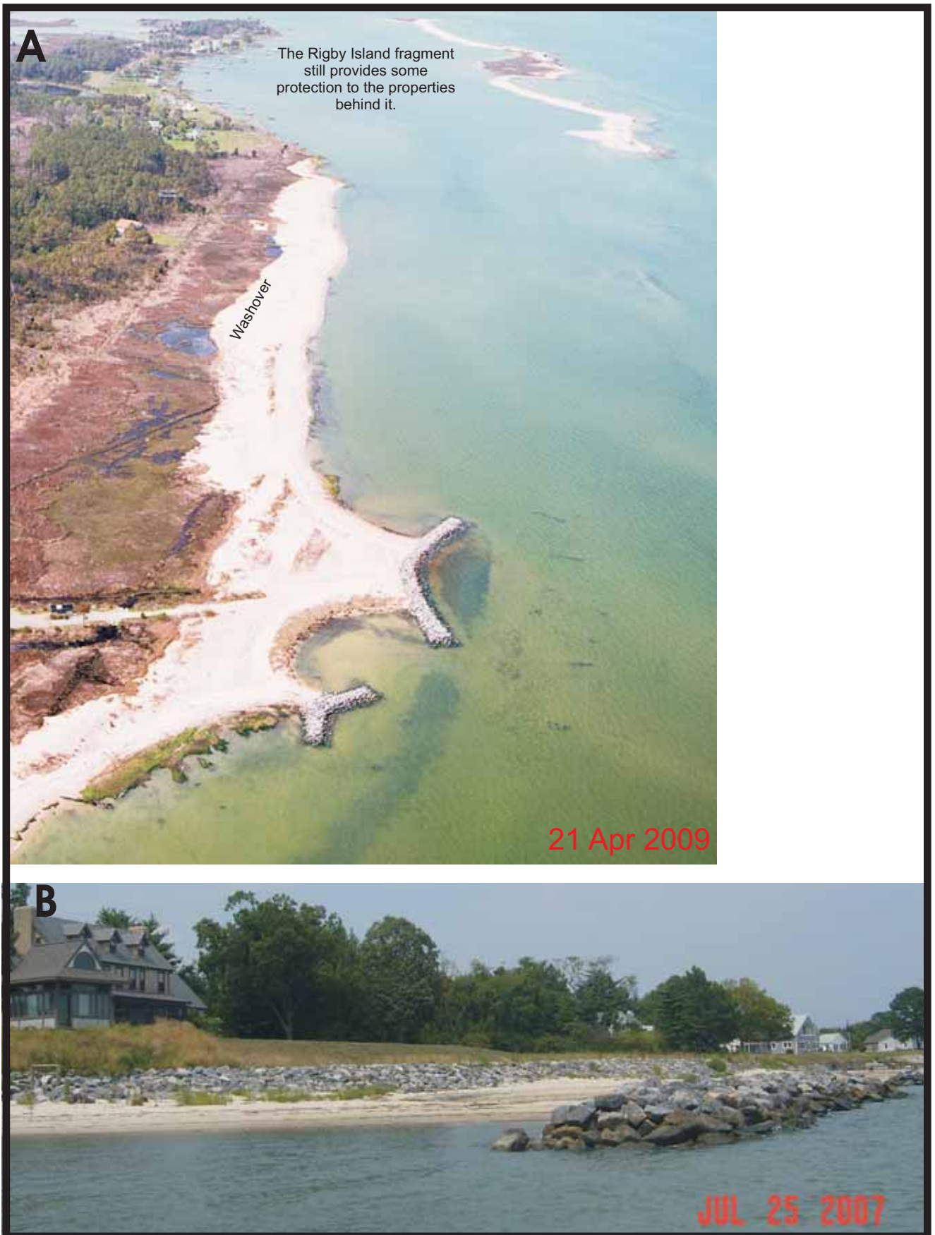
Figure 2-8. A) Breakwaters built on Chesapeake Bay at Festival Beach, Mathews, Virginia and B) breakwaters built on the York River in Gloucester, Virginia.
