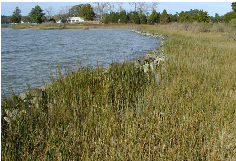
A shallow nearshore zone can support marsh growth but the wave exposure requires a marsh sill to protect the plantings from wave energy. If the wave exposure were low, a temporary bio-log would be sufficient.
